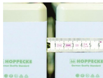
Fig. 5-14: 10 mm clearance between the batteries
